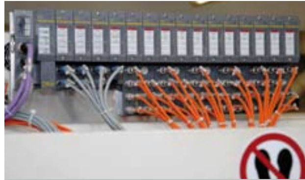
FRIMO uses Turck's I/O system BL67 also for transmitting high frequency signals Page 18
